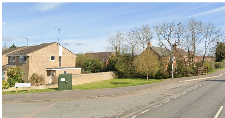
There is already a DSLAM cabinet on this verge, installed 2014
