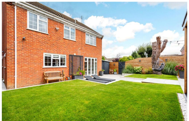
Rear elevation and part of the garden area
