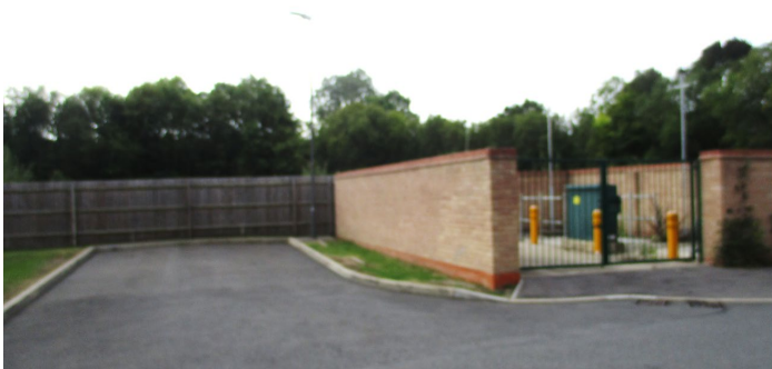
The site access from Foundry Drive, sewage pumping station on the right These photos were taken in 2022 for the previous application
