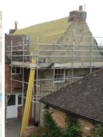
The work being done in April
