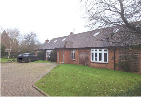
The existing bungalow
