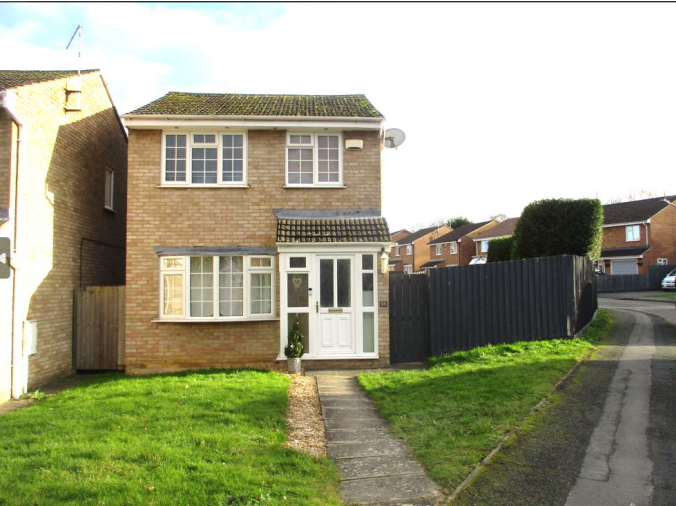
The front view of No 33. The grassed area to the front of the house and close-board fence is not included in the red line boundary on the drawings, but the grass between the back fence and the driveway is.
