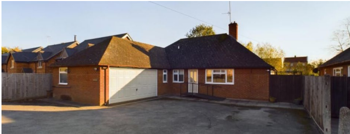
View of front of existing dwelling
