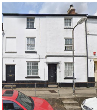
No 9 (left) & No 8 Well St.
