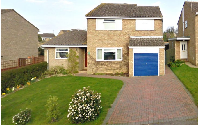
Front elevation. The public path is on the left, between the hedge and the fence with the trellis
