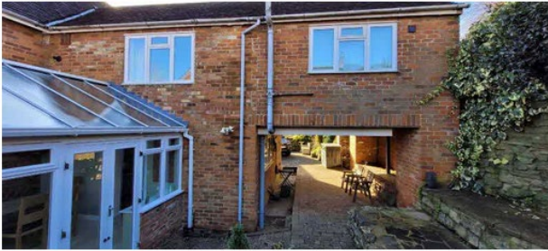
Side (northeast) Elevation
