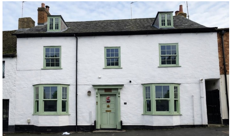
Street elevation (applicant's photo)
