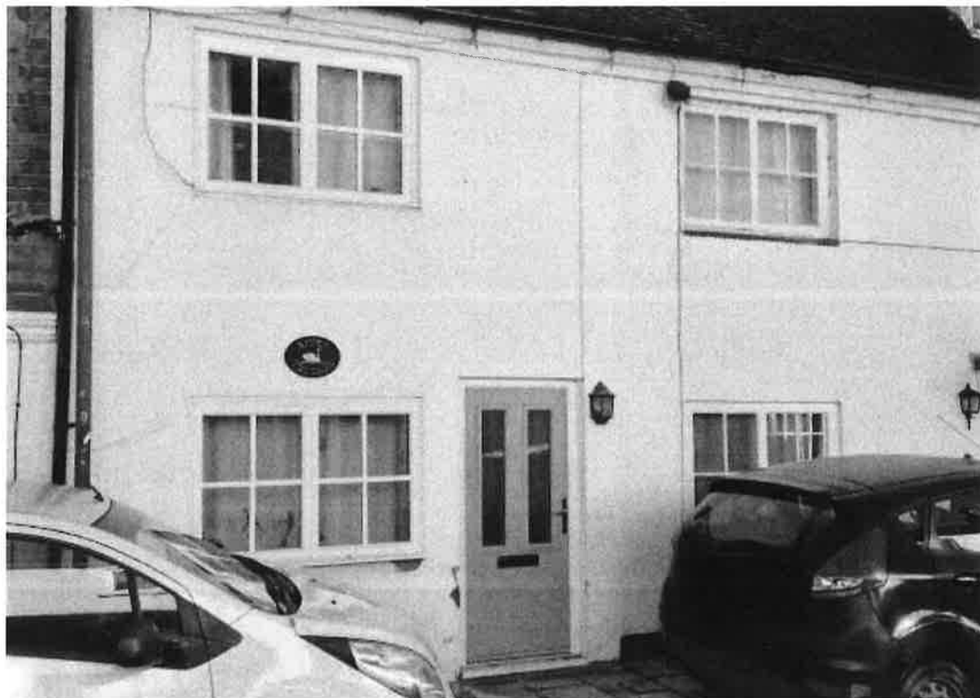
Front elevation with replacement windows – September 2025
