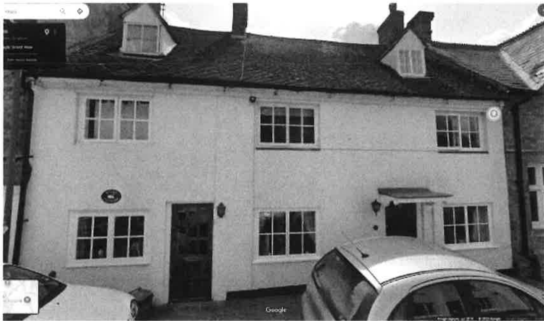
Front elevation of 50 Well Street – July 2018 courtesy of Google Street view.
