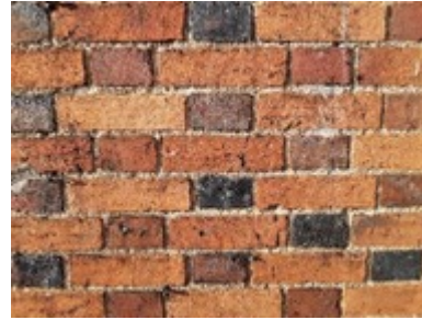
Flemish bond with vitreous headers
