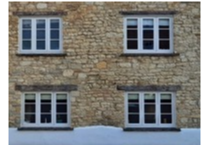
Coursed limestone rubble
