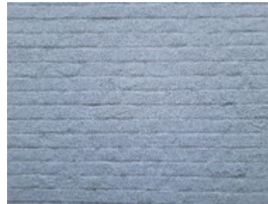
Painted English bond brickwork
