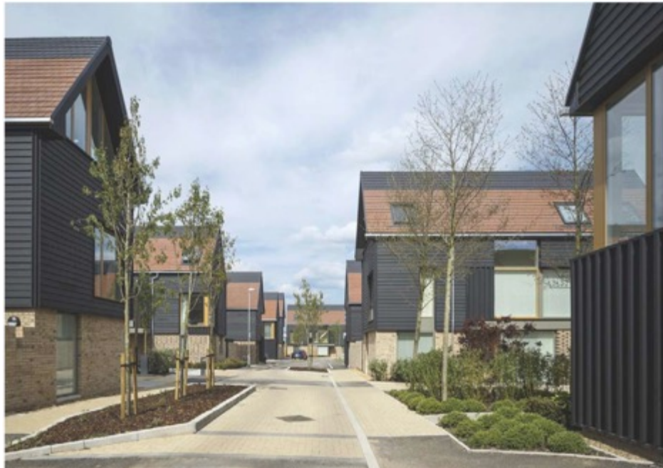
Example of use of physical features and planting as chicanes to slow traffic speeds and prevent vehicle access, National Model Design Code
