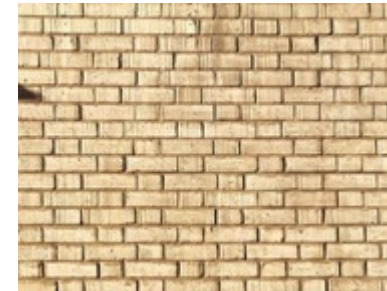
Yellow bricks laid in Flemish bond
