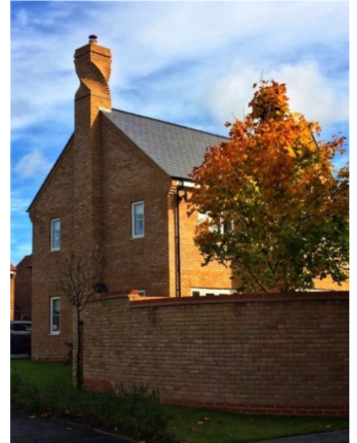
Modern interpretation of the historic chimney erected in 2012.
