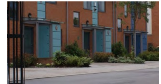
House frontage bin storage good practice example. (Image credit: Oxford County Council Street Design Guide.)
