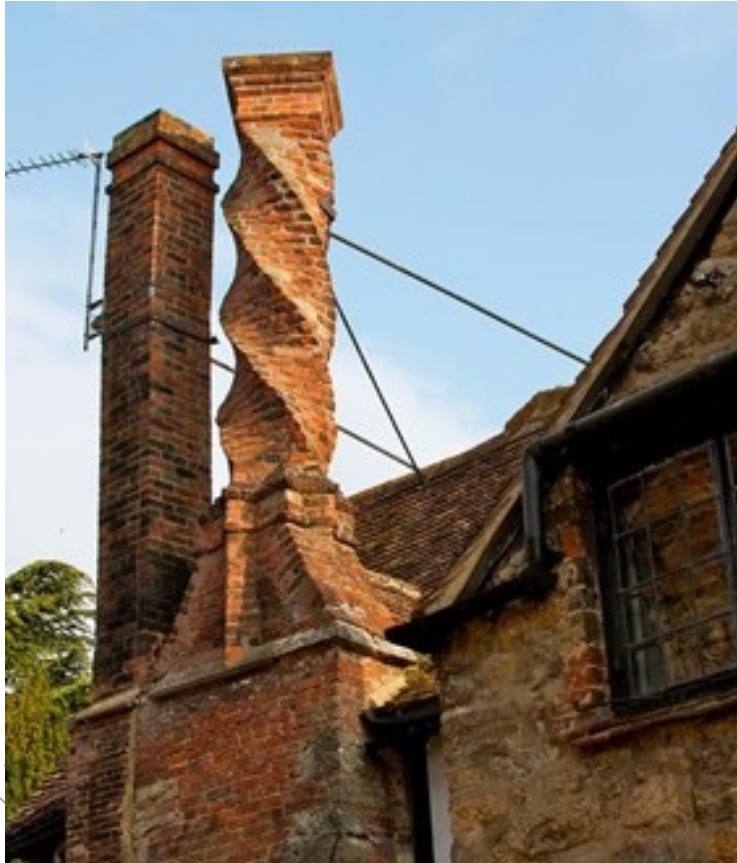
Historic twisted chimney attached to Grade 2* Listed Building and dating from the 16th century.
