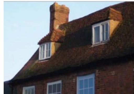
Dormer windows positioned away from ridge
