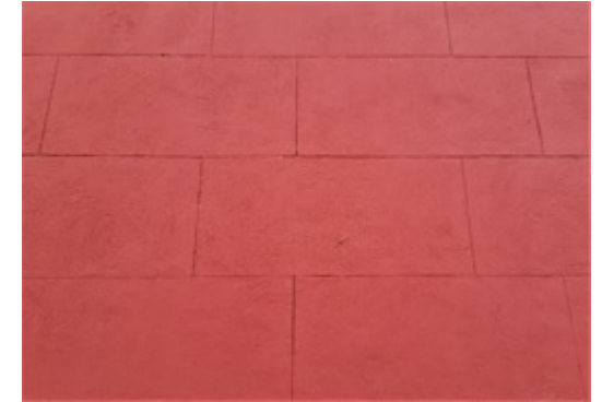
The incised masonry pattern
