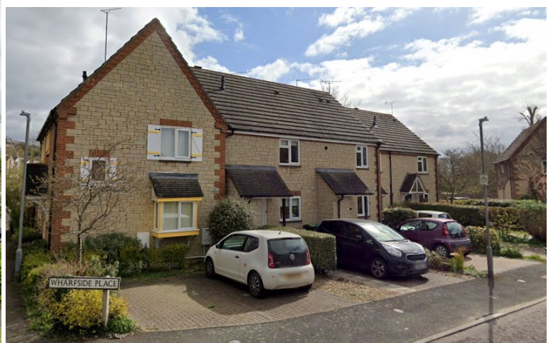
Flank elevation of No 1 and fronts of Nos 3-9 (odd numbers only)
