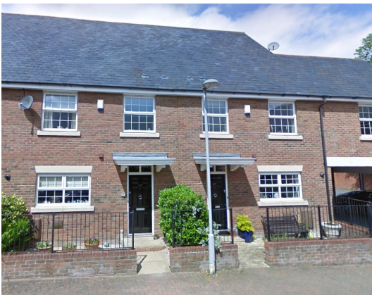
Front view of Nos 25, 27 and parking court archway
