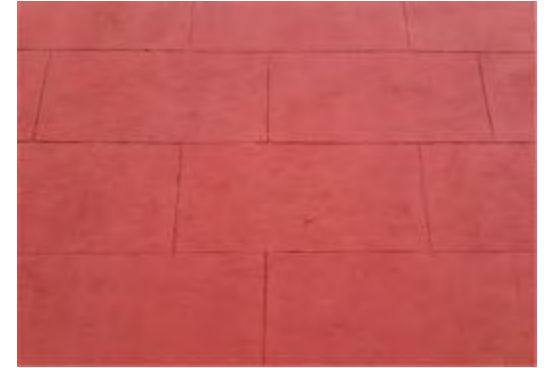
The incised masonry pattern
