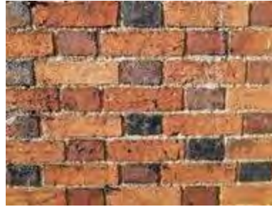
Flemish bond with vitreous headers
