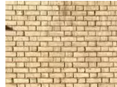
Yellow bricks laid in Flemish bond
