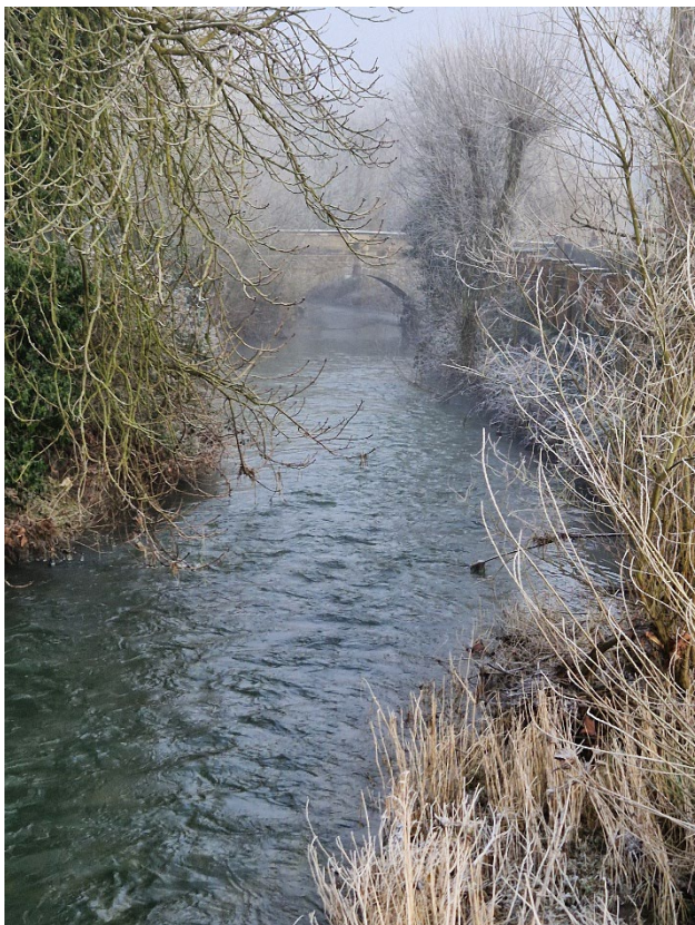
1 Ford Street Bridge looking towards Bridge Street
