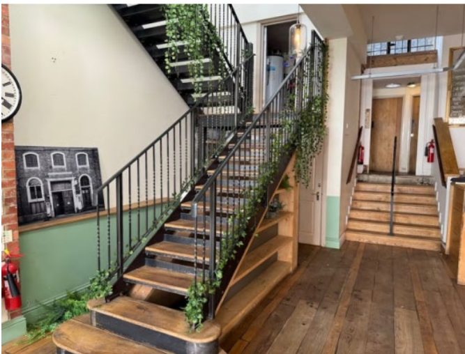
The modern staircase and plant room; the upper flight is to be removed and the gap made good
