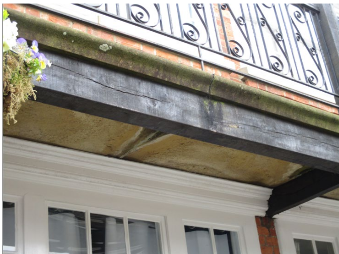
Underside of balcony showing damage and lamination due to damp (23/4/24)
