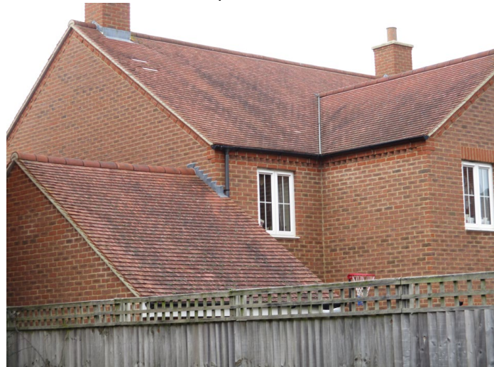
Rear of house and garage from Catchpin St. flats' carpark
