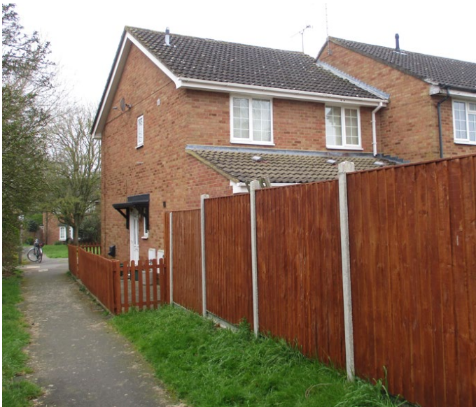
General view of side and rear of house
