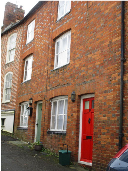
Nos 9 (red door) and 10
