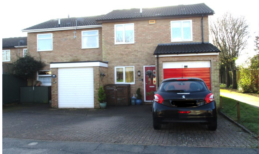
Nº18 (red door) and Nº20 (16/2/24)
