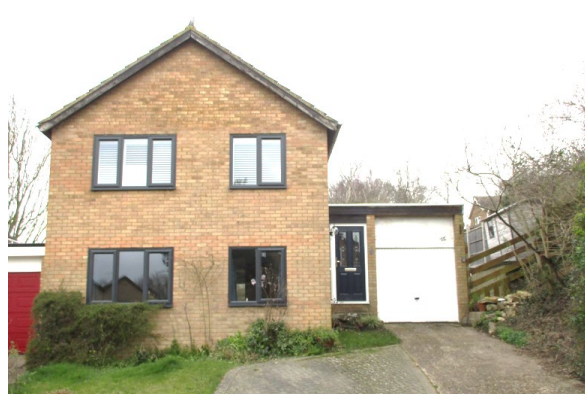
The front view of the house
