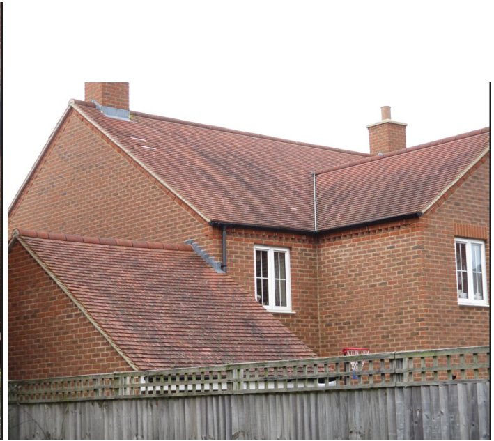
Rear of house and garage from Catchpin St. flats' carpark
