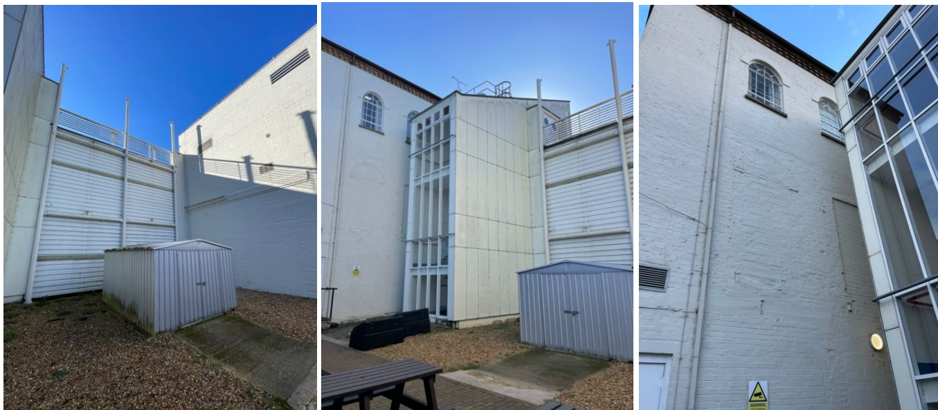
Location for the new stairwell and the shed to be demolished and the existing stairwell/lift shaft in the other corner of the courtyard with (just visible under the render) the infilled window next to it, below the remaining glazed one (see drawing below right).
