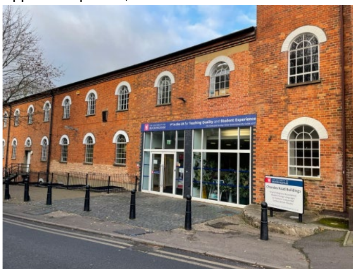
Station Road frontage; the window over the righthand part of the entrance replaced a large boarded-over gap which may have housed a gantry; a window from the rear of the building was used, to match the others.
