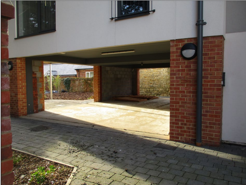
The undercroft area (left) and the existing view to the garden. The columns support the first floor terrace/balcony
