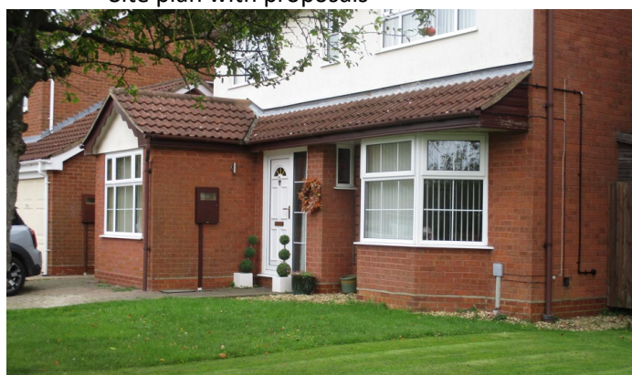
Existing former garage/porch/bay window
