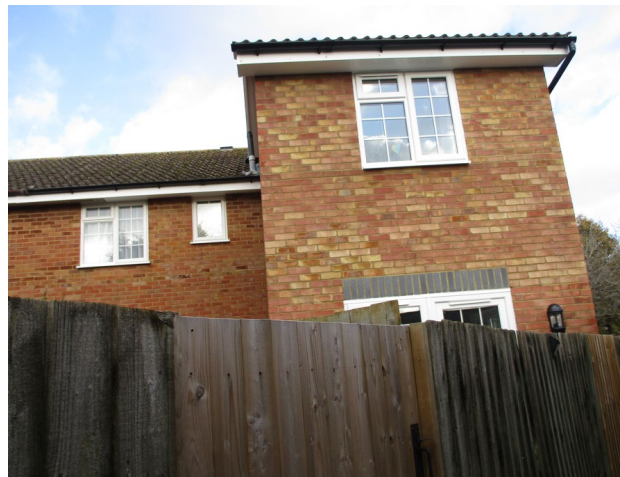
The rear view from the public path. The fence dividing the two garden areas can just be seen in the centre
