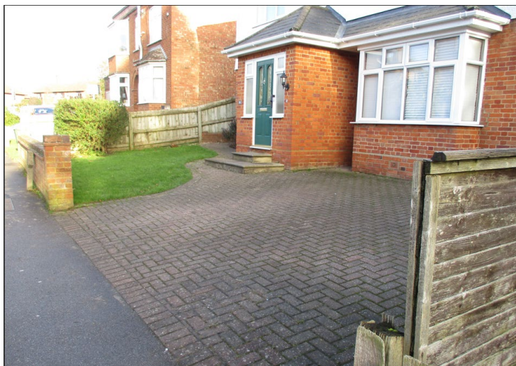
The front garden as existing (22/1/24). Presumably the rest will be paved to access the proposed cycle racks(drawing above left)
