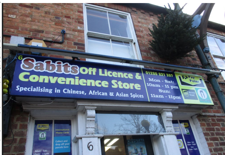
The fascia sign (striplight over) and scrolling panel (over door)
