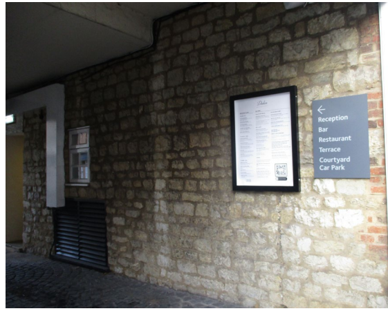
These are the existing signs in the archway
