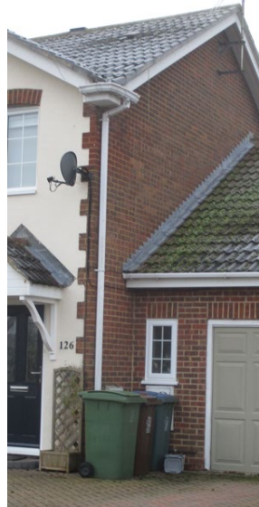
The angle between house and garage where the extension is proposed (30/11/23)
