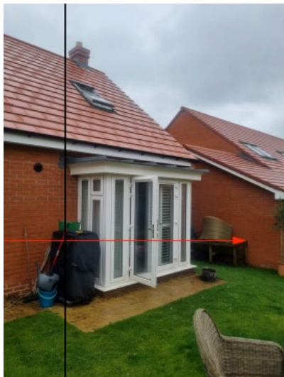
Existing projection at rear of kitchen
