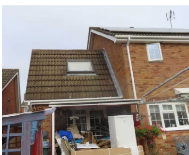
(Photo 4) Existing garage roof- rear
