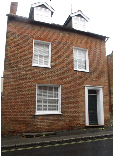
Front (note basement window)
