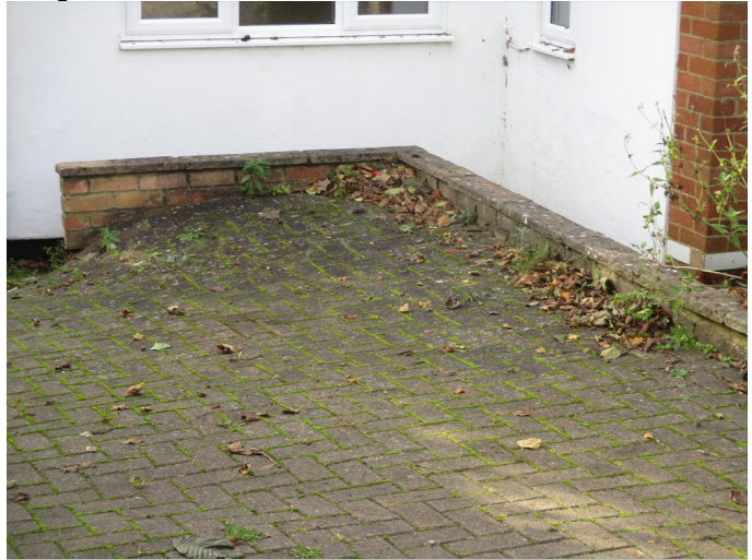
Small bay to left of front door
