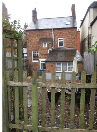
Rear from parking bay
