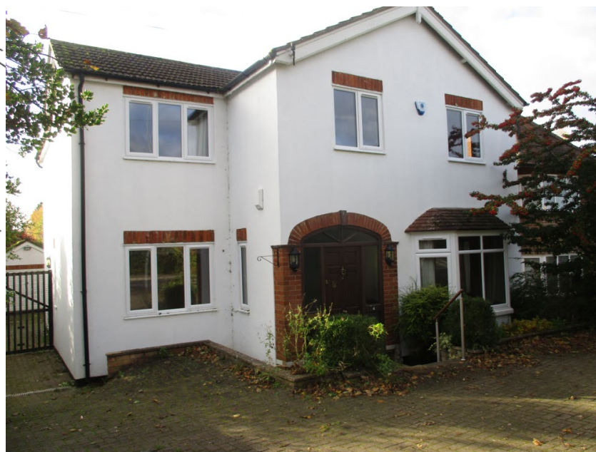
The front of the house (15/11/23)
