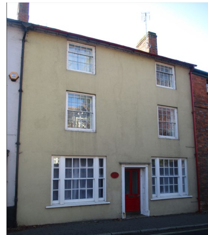
Front of building 11/11/23
