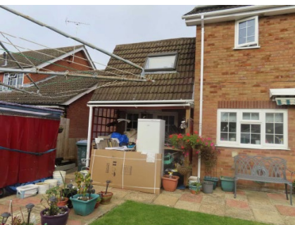
(Photo 3) Existing garage- rear
