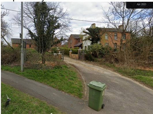
Outbuilding (L, behind tree) and farmhouse (R)
