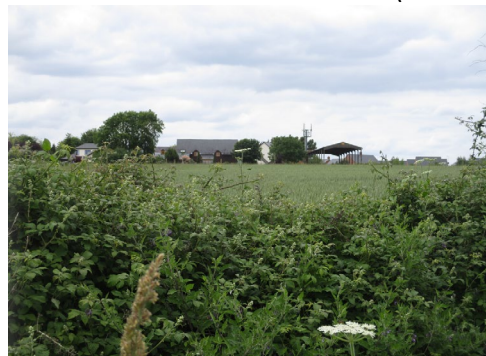
View of Benthill from the public bridleway The open-sided shed is to be demolished
