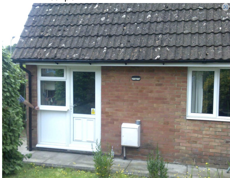
Applicant's photo of existing rear wall
