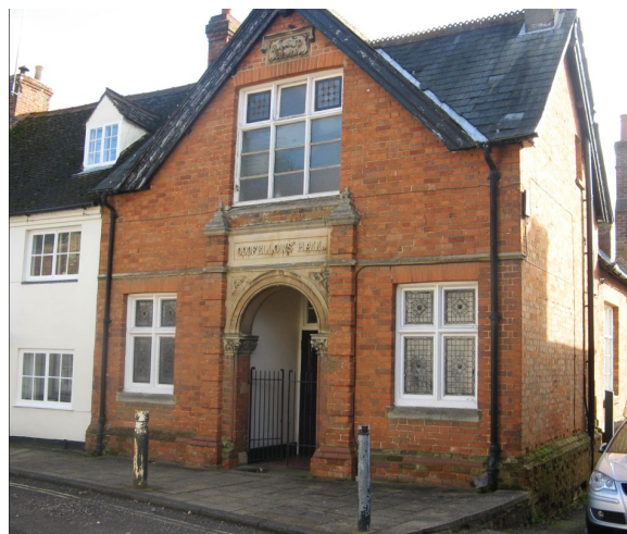
The room on the left of the front door is the bin store
