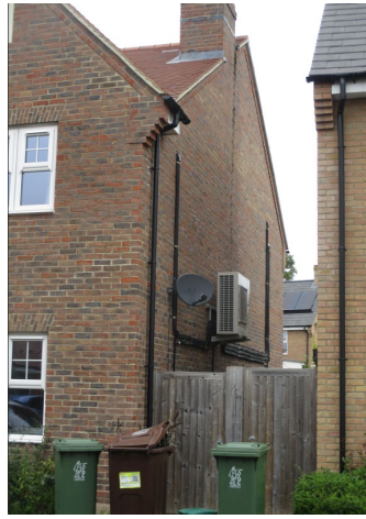
Installation on side of house (No18 on right)
