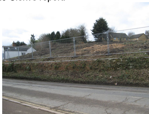
Existing retaining wall below proposed access
