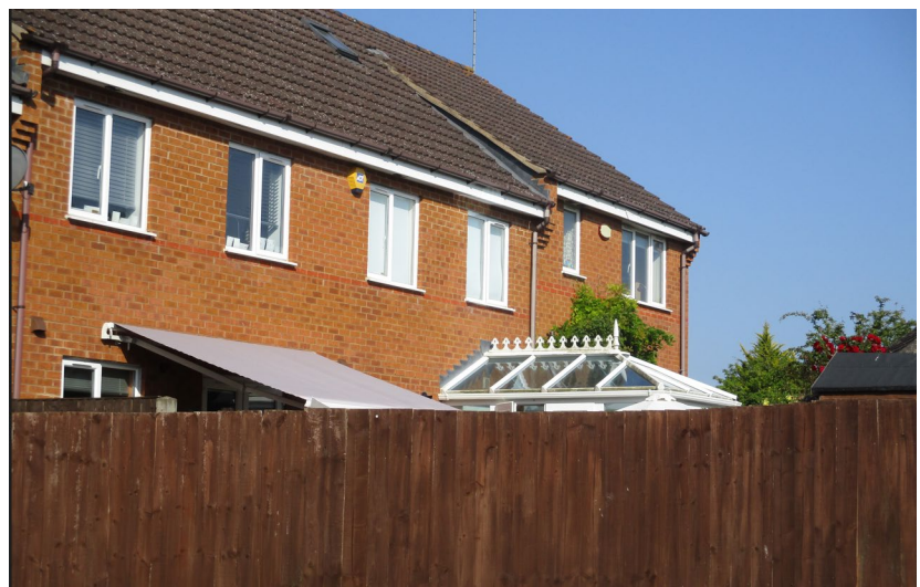
The existing conservatory, from the parking court beside No 47 (9/6/23)
