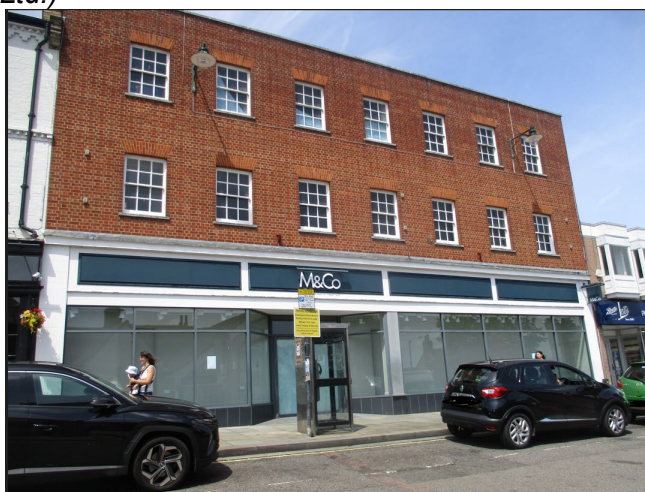
Front of building 23/6/23
