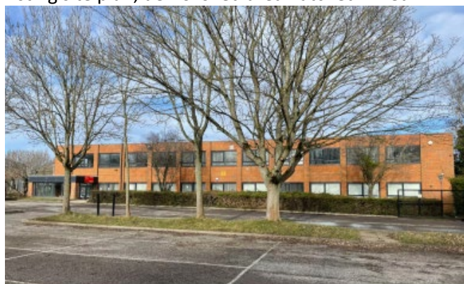
The office block to be retained
