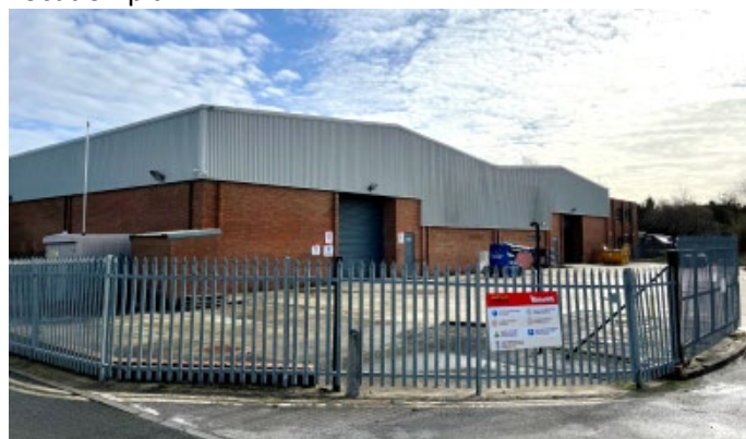
Unit C before demolition
