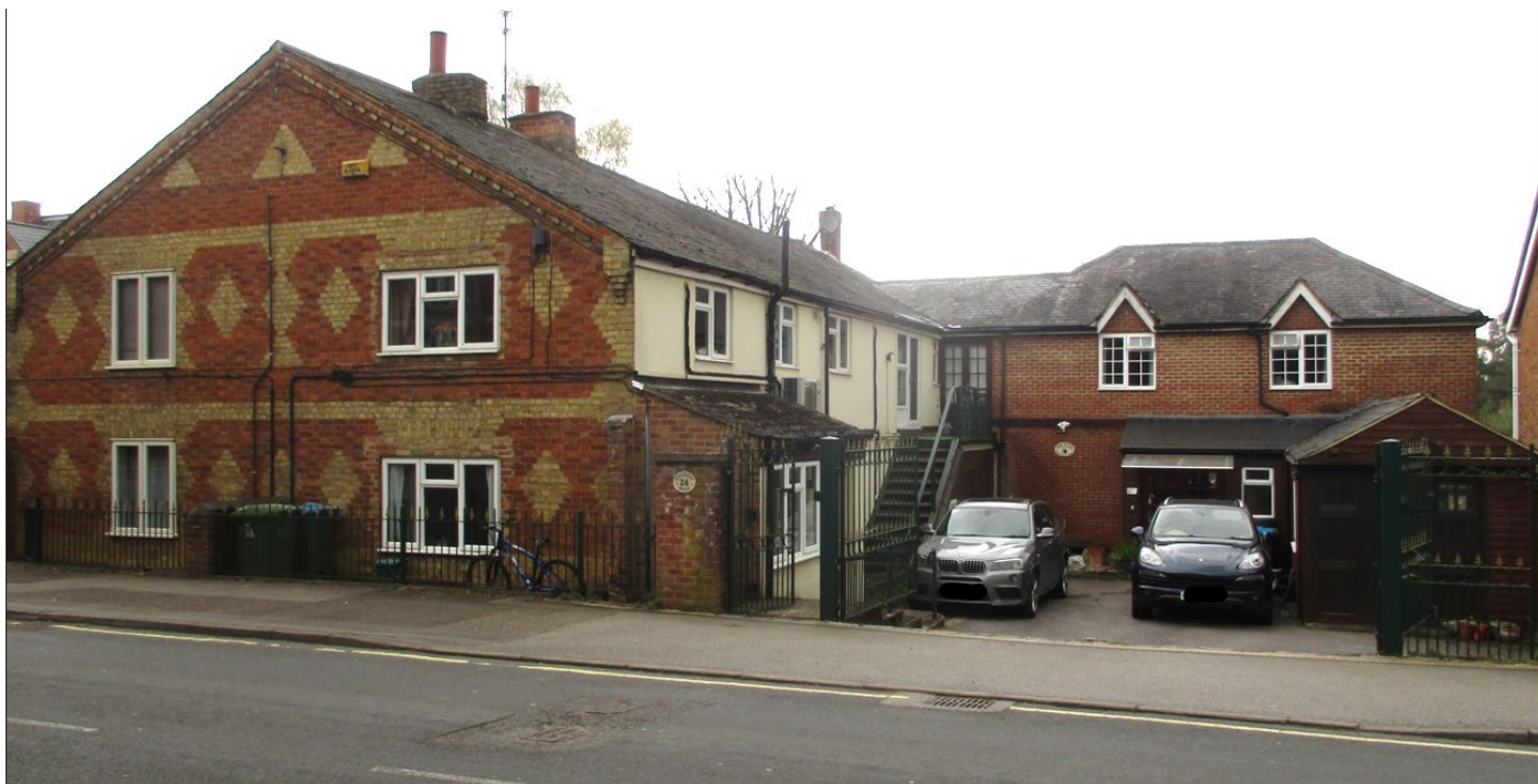
№ 25 ↑ ↑ № 24 from here to right hand side of photo ↑ rendered building Units 2-4 ↑ Unit 1 & garage
