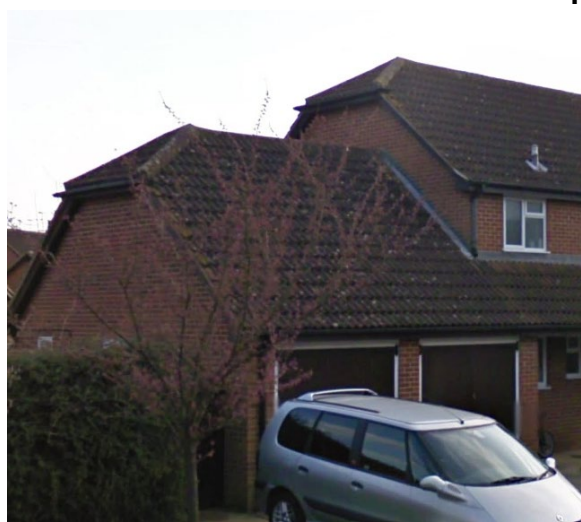
The hipped gables on the garage and house roofs
