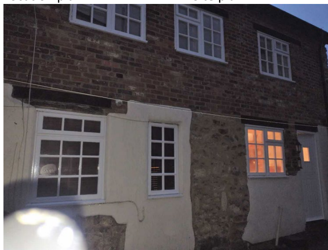
These are the windows and door to be replaced
