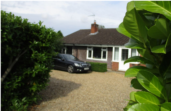
Front of existing bungalow – southern end
