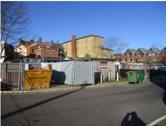
View from southeast towards rear of Market Square
