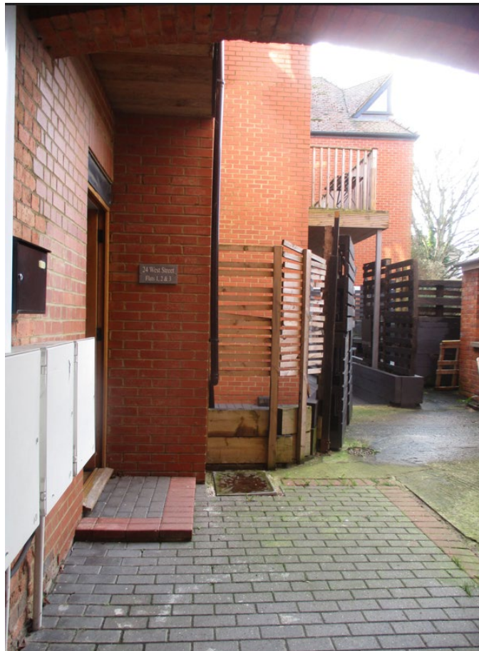
View from arched passage of remains of courtyard with entrance to existing flats A, B & C on left
