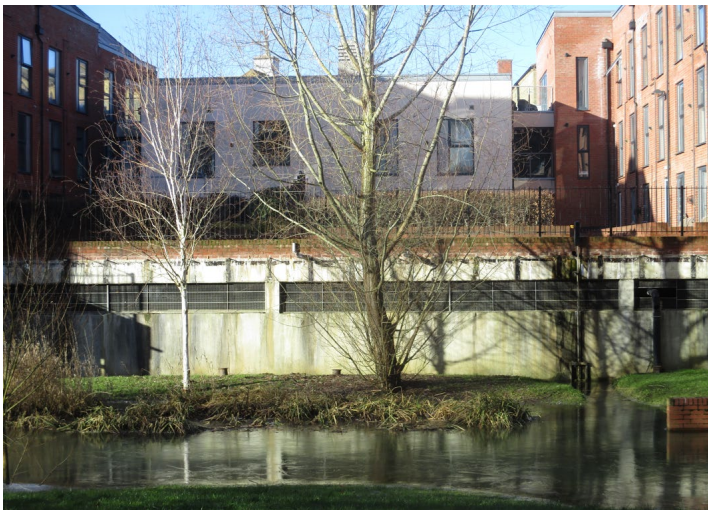
View of the floodwall from riverside path, across the lake
