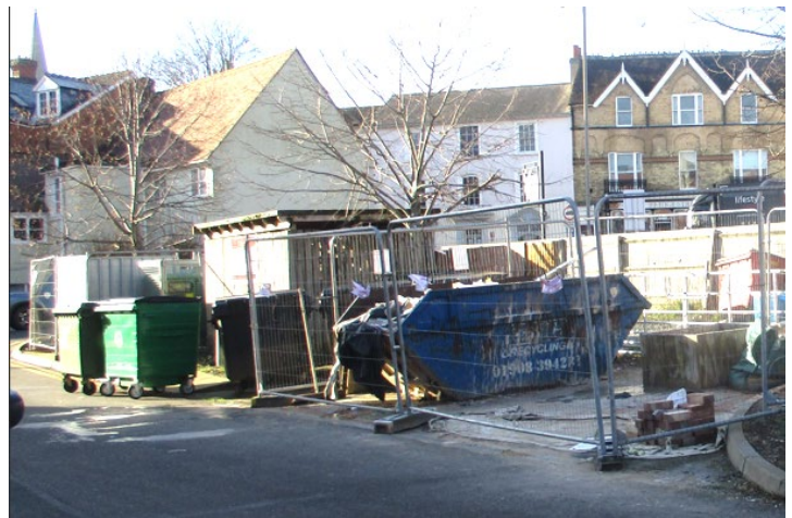
View from northeast towards Bridge Street shops
