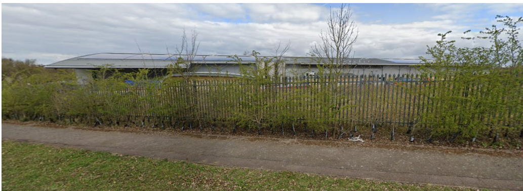
The site and existing factory
