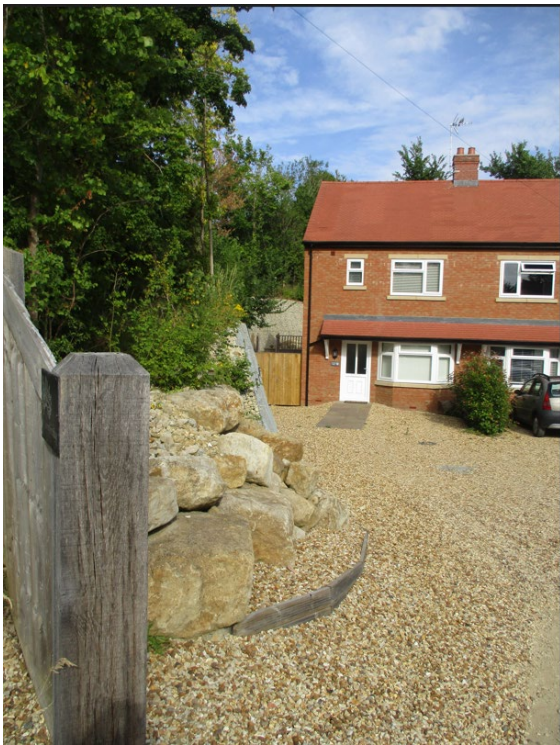
Cherry Tree Cottage – site is above gabion wall at rear
