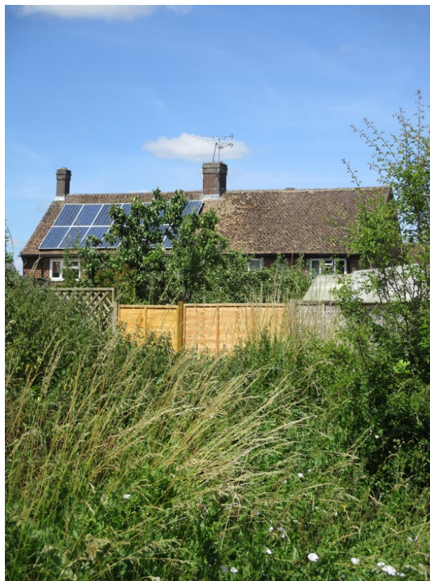
Rear view from disused parking court (№11 on the right)
