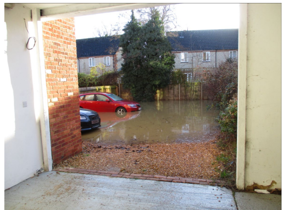
Parking yard at The Villas, Stratford Road Taken c.11am, 24/12/20
