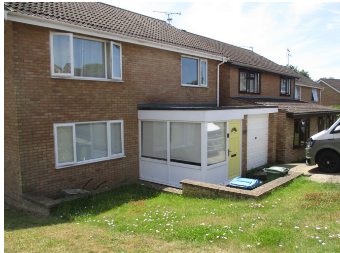
The front of No1 (and No3 behind) : the difference in level can be gauged from the bins in front of the porch.
