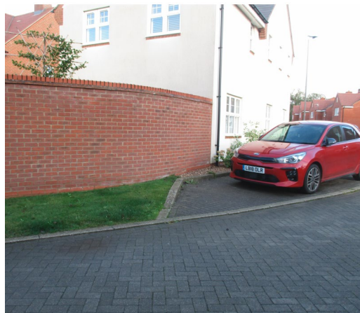
Photo of rear boundary wall
