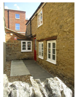
Site to be infilled
