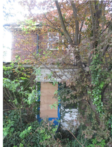
The side of the house from the public path with the flat-roofed element
