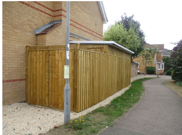
Fence to front and side (26/8/22) and shed
