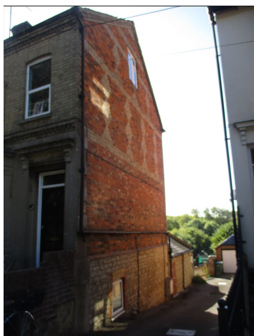
Alley between Nos9 & 10
