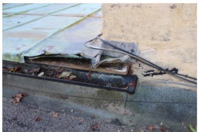
Existing Copper Roof Eaves - East Lodge
