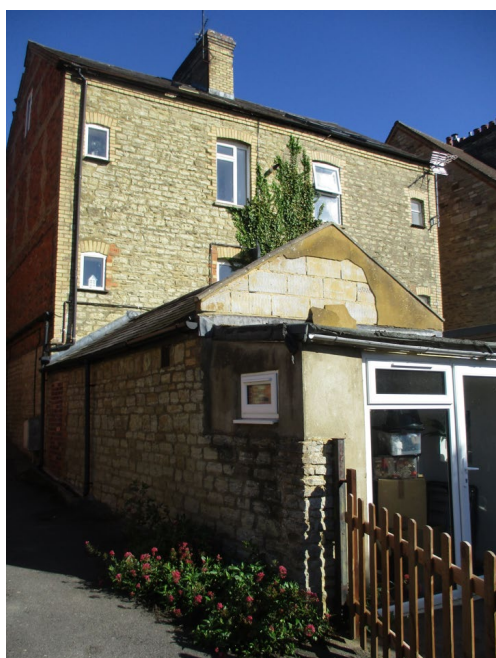
Rear view of Nos9 (left) and 8 (right)
