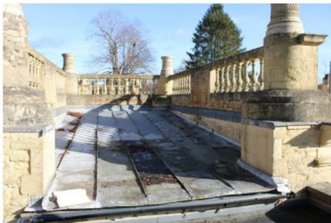
Existing Copper Roof- West Lodge
