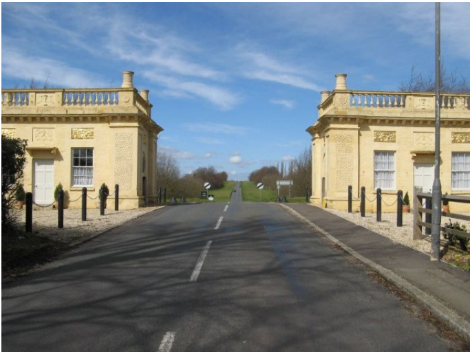
West and East Lodges and Stowe Avenue
