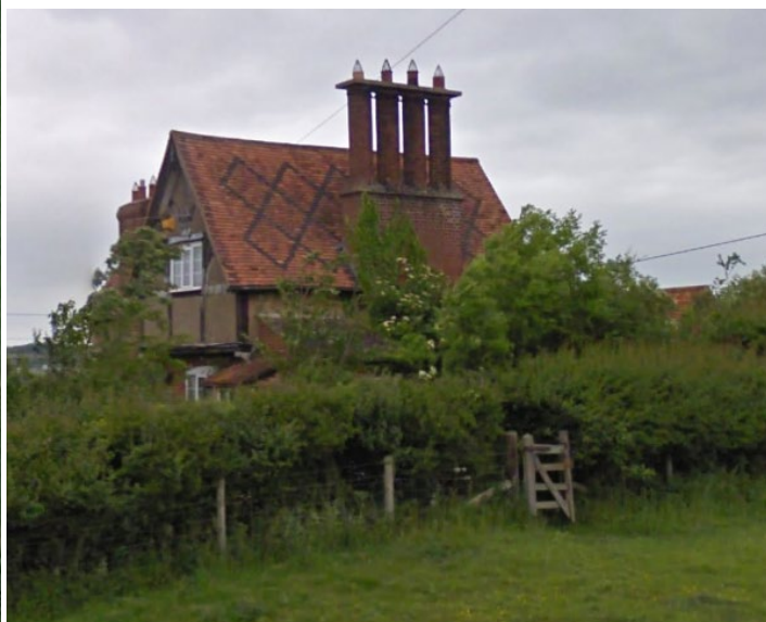
View of No. 2 from farm lane
