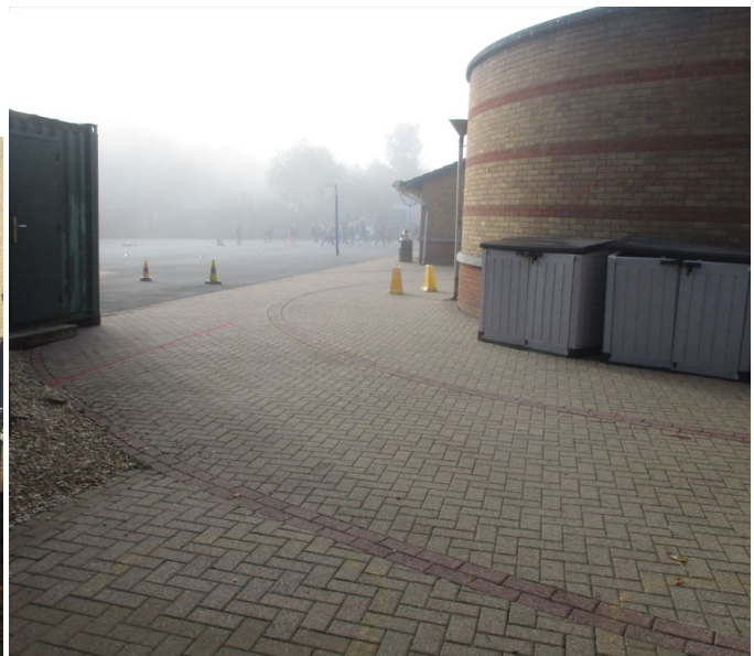
The site for the heat pump installation (18/10/22)
