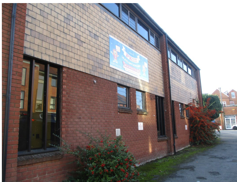
2 storey block looking towards Well Street access
