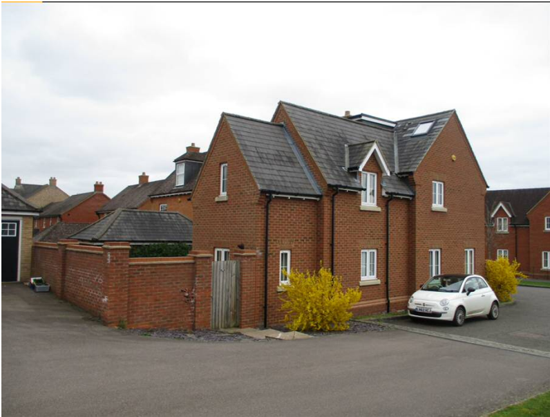
Side/rear view of 26 Shetland April 2021
