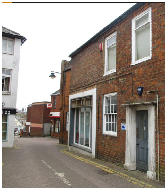
Door at right is access to 23a, first floor flat
