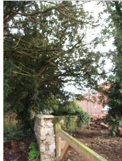
The yews overhanging the boundary wall
