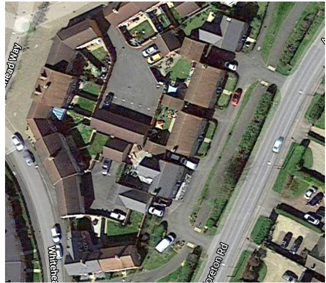
Google satellite view pre-dates addition of dormers & rooflights
