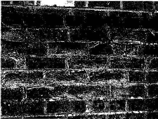
Close up of brickwork from play area side.
