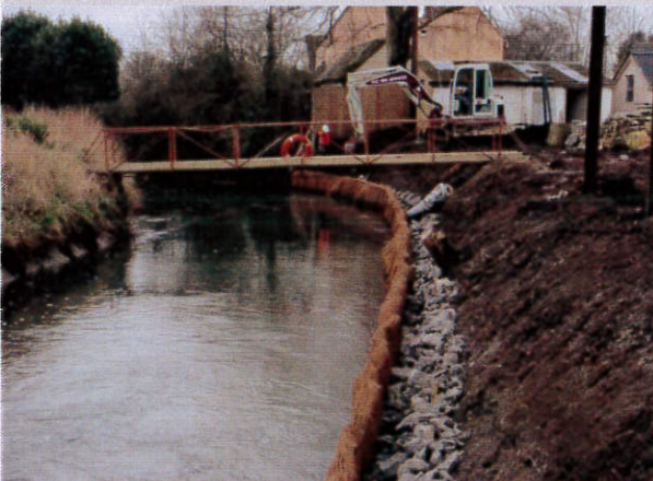
During construction – Geotextiles are placed against posts and the structure is filled with limestone and finished with topsoil and native planting.
