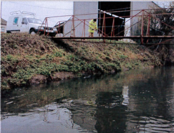
BEFORE summer 2010- Eroding steep bank on an outside meander on the River Sheppey due to undercutting and bank slips.
