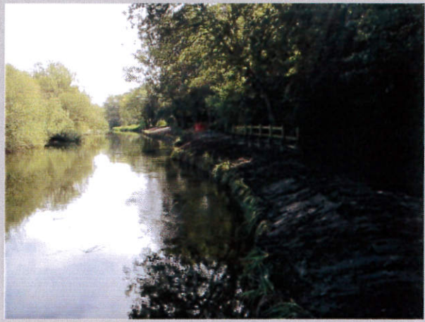
Post construction – Bank line stabilised with a coirnet revetment, planted with site won plants and line of footpath restored.
