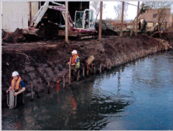
During construction – Line of sweet chestnut posts being driven to form new toe of bank.
