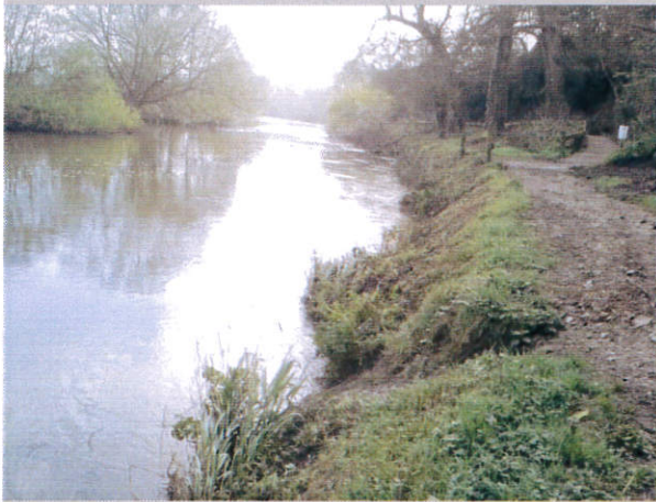
Before construction – Banks has eroded and is collapsing into river de-stabilising a footpath.
