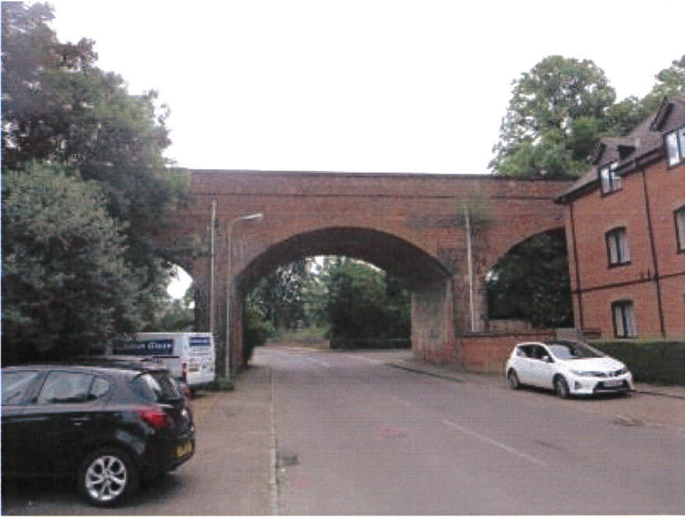
Photo 2: General view of South elevation
