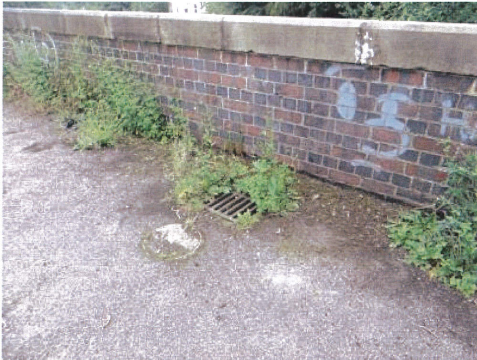
Photo 15: Drainage gully at top level.
