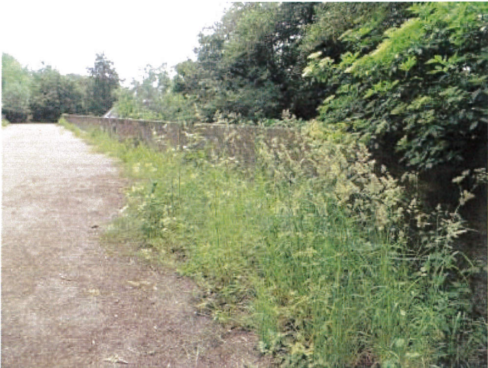
Photo 15: Vegetation growth along verge.
