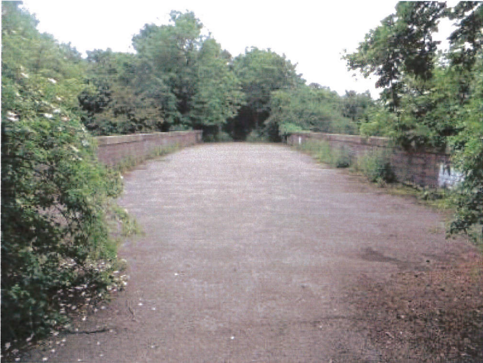
Photo 4: View over bridge from East
