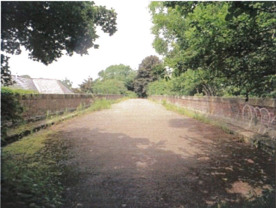
Photo 3: View over bridge from East
