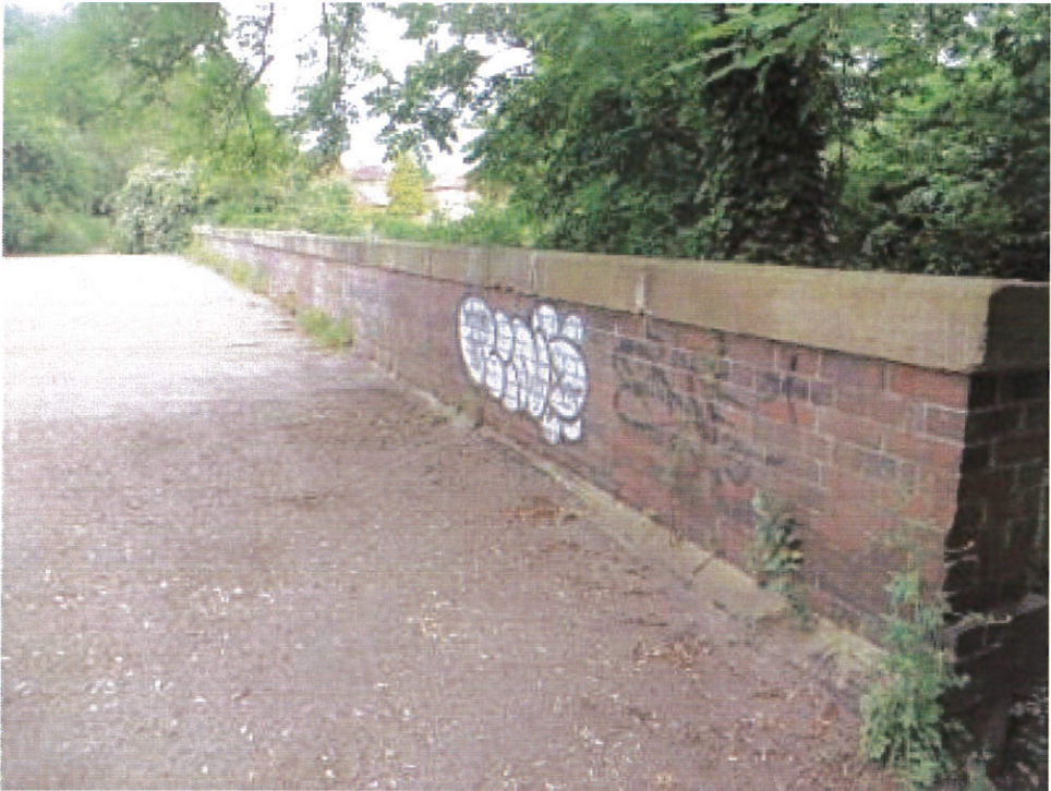
Photo 3: View over bridge from West
