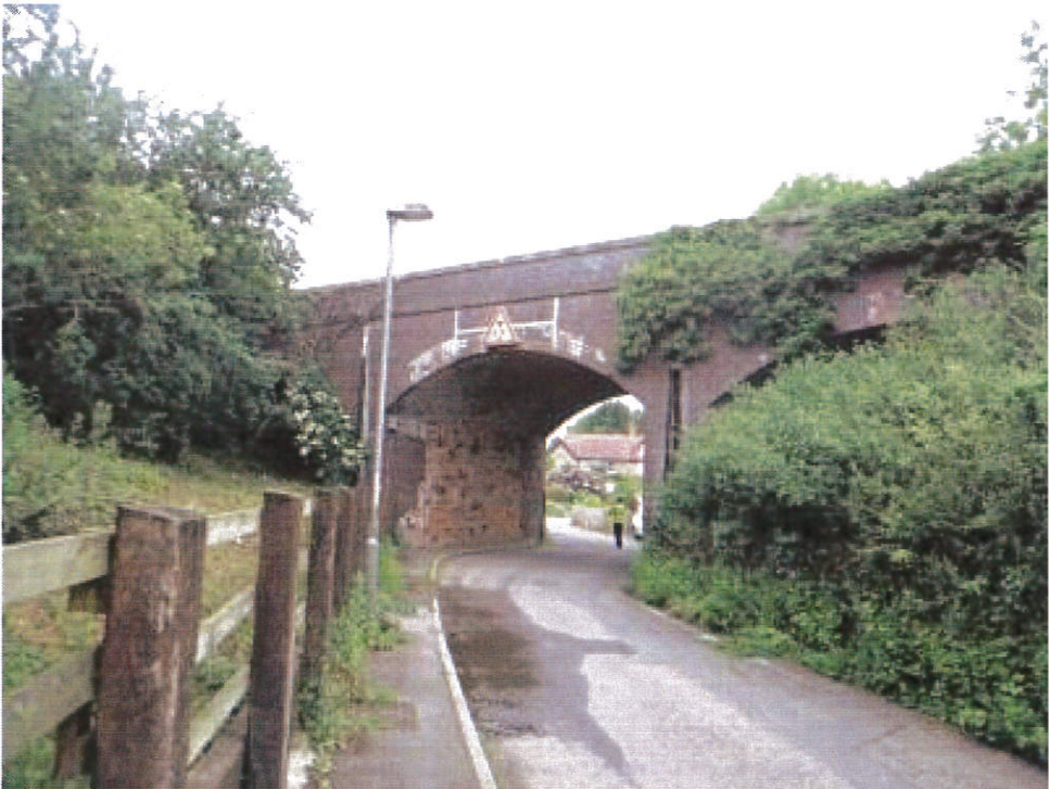
Photo 2: General view of South elevation
