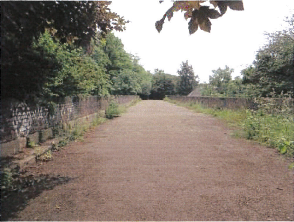
Photo 4: View over bridge from West
