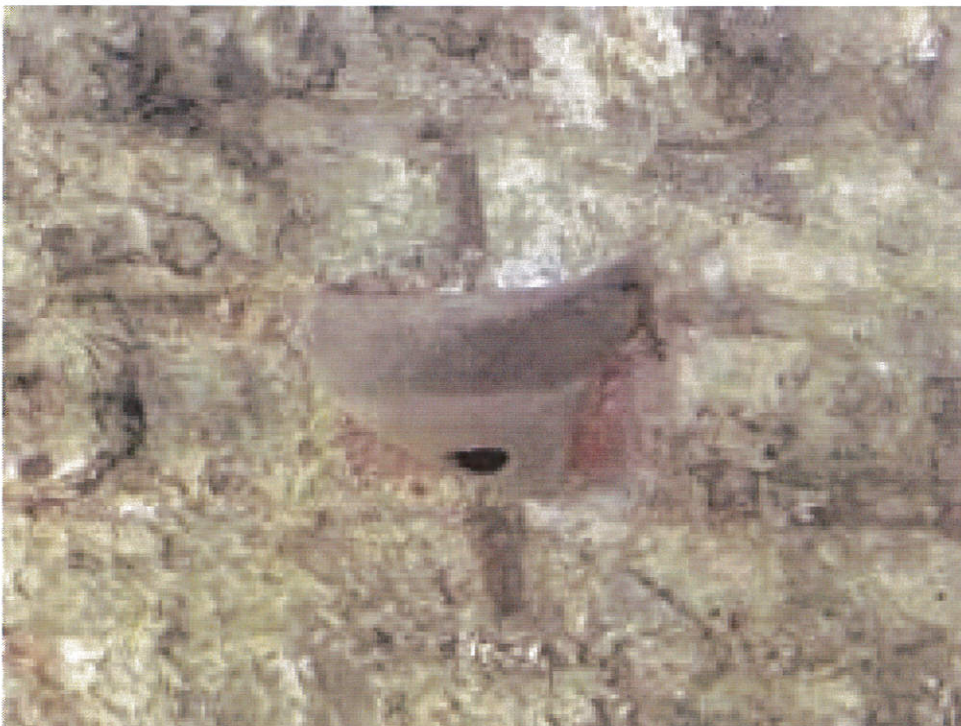
Photo 16: Climbing handhold fixing.
