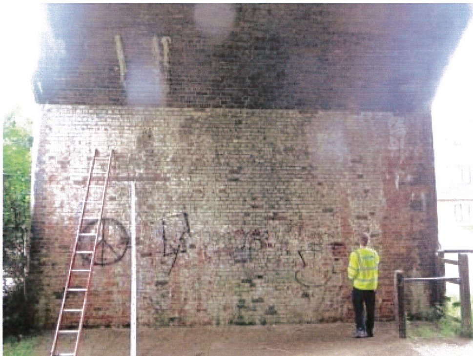
Photo 8: West elevation of pier 2/3.
