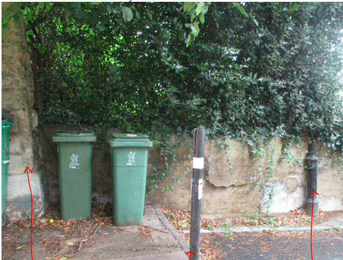
Church gateway pier
