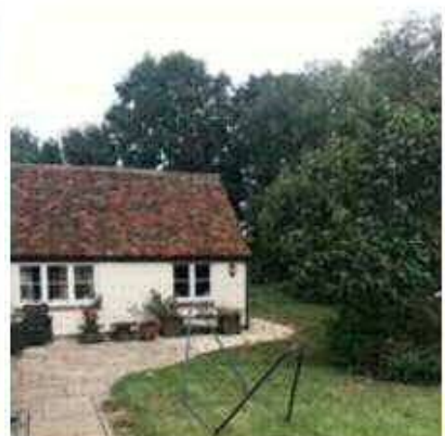
The single storey extension from the South West
