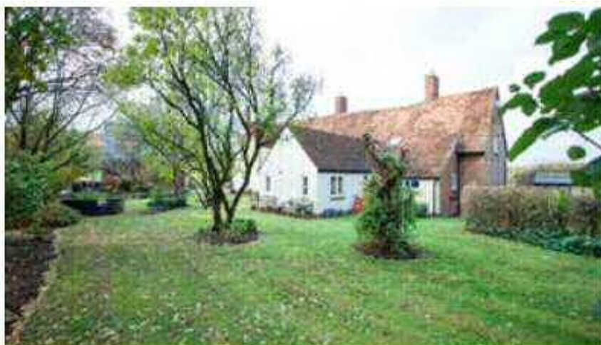
View of the rear of Rose Cottage looking from the East/South East including the 1990's single storey extension and the existing utility room under the cat slide roof
