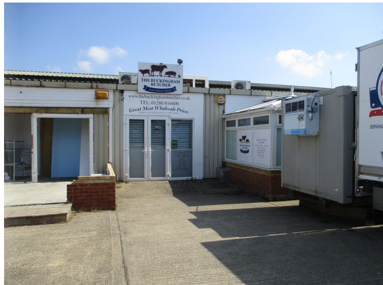
Existing front of Units 9 & 11 (24/4/22)
