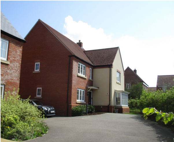
House from northwest (photos taken 24/4/22)
