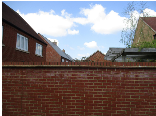
Rear of house, side wall, and garage roof behind loggia
