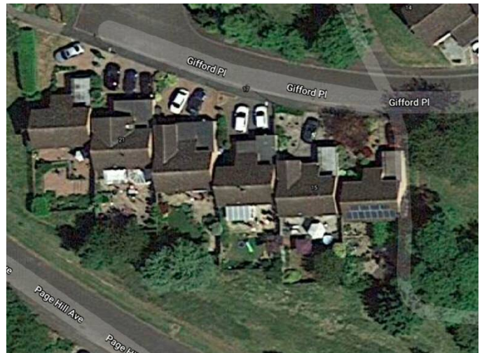
Aerial shot - No 17 has 2 white cars in front, and large conservatory at rear (to be demolished)
