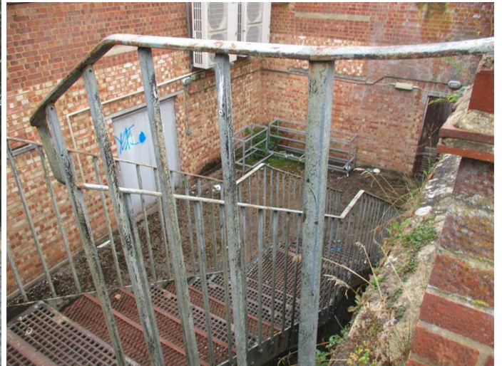
The basement door served by the fire escape
