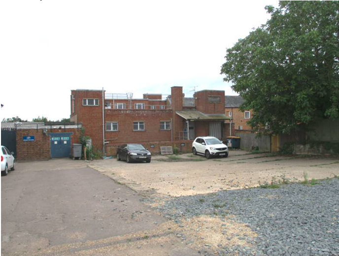
General view of rear of building from yard
