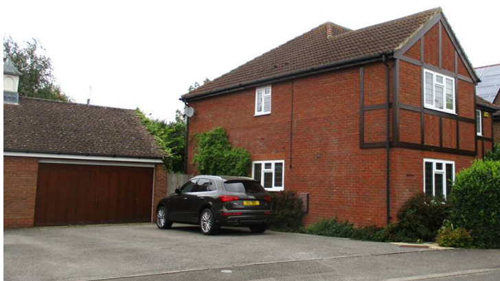
Front of house, double garage and hardstanding (25/8/21)
