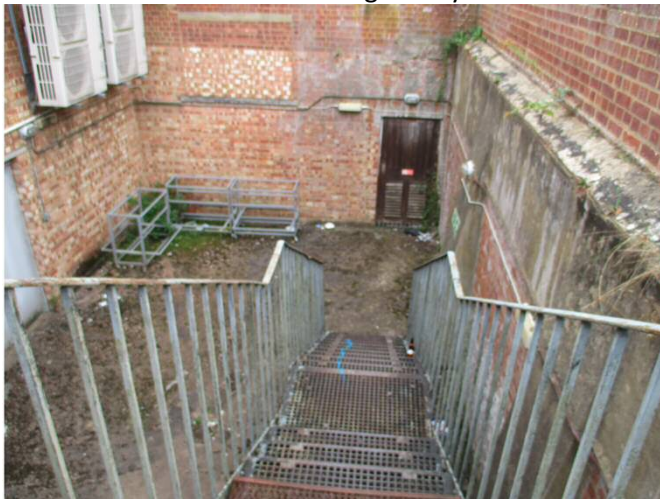
General view of basement area from ground level walkway
