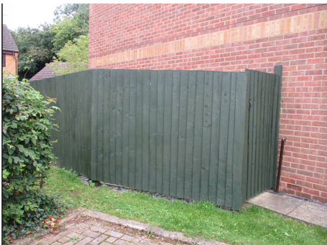
Gate and angled part of fence is to form bin storage area; Side extension proposed behind remaining part of fence
