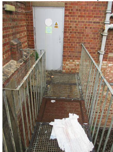
Ground floor fire escape and walkway to parking area
