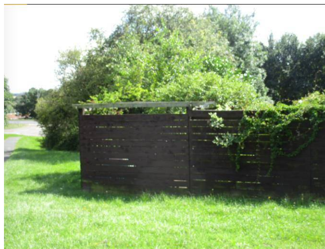
Rear corner – existing pergola visible (10/8/21)
