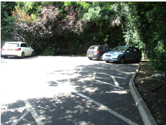
Cars in the two end bays; one bay and the disabled bay with side hatchings on the northern edge. There are two further bays behind the photographer
