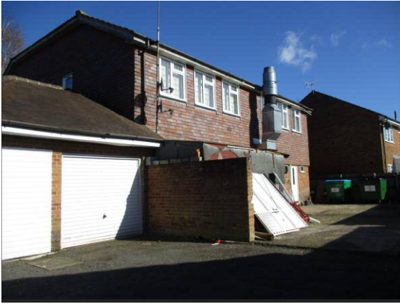
Rear elevation and garage
