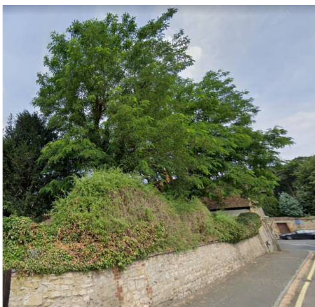
View from School Lane (2018) (Google)
