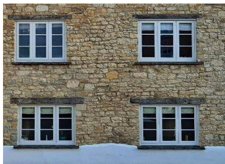
Coursed limestone rubble
