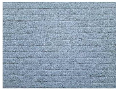
Painted English bond brickwork
