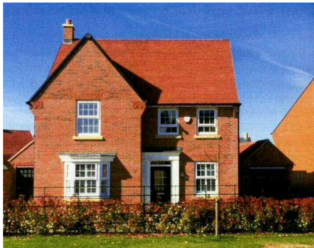
New dwelling within Lace Hill designed and built to reflect the local distinctiveness of Buckingham.
