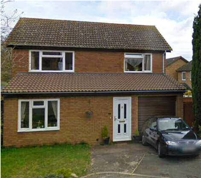
The adjacent №9 Boswell Court (floor plans are reversed); №11 will be similar, with rooflights over the door and lounge window.
