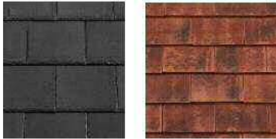
Natural slate tile and plain clay tile
