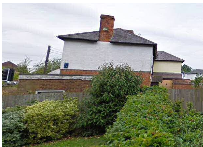
Side view of No 25 from Bernardines Way; No 23's extension visible behind shed
