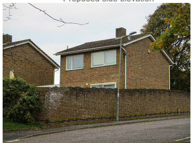
Rear view to gauge how much extension will show over wall
