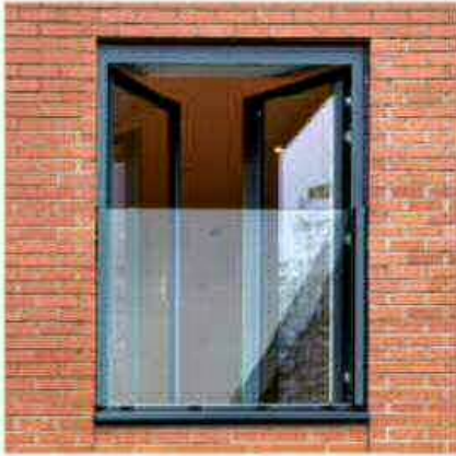
2 New Juliet balcony overlooking woodland with glazed balustrade
