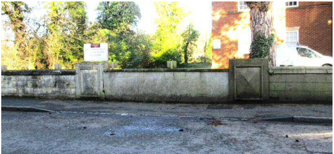
.... and there are still two (without capstones) opposite, outside Barham Lodge
