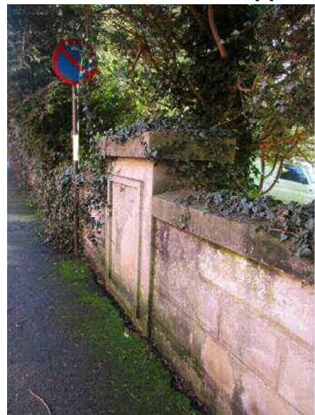
view of pillar showing thickness
