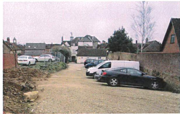
Top of site looking towards West Street archway
