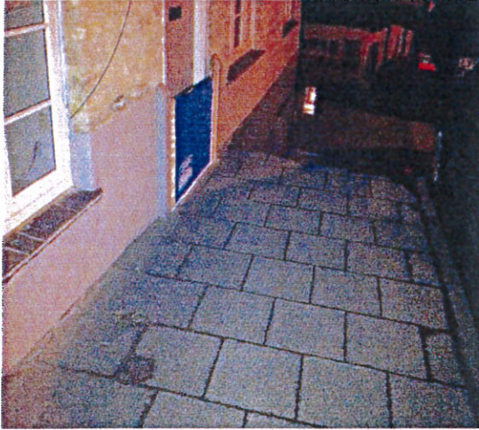
Ford Street, Buckingham at 12.15am, 10 th March 2016. Property level flood protection board (blue barrier) in operation (photo provided by Buckingham Flood Action Group).
