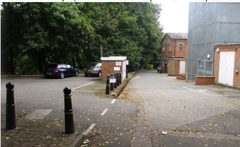
The car park entrance and road to the rear yards. The prayer room will be to the left rear where the cars are. The small brick building behind the row of bollards is the substation; the marked parking bay in front of it is not on the drawings. The debris netting is on the rear section of the main Chandos Road Building building, the central yard is between this and the rear brick building (the smaller white door is the portacabin); the maintenance yard is behind the further brick building where the green skip bin is.
